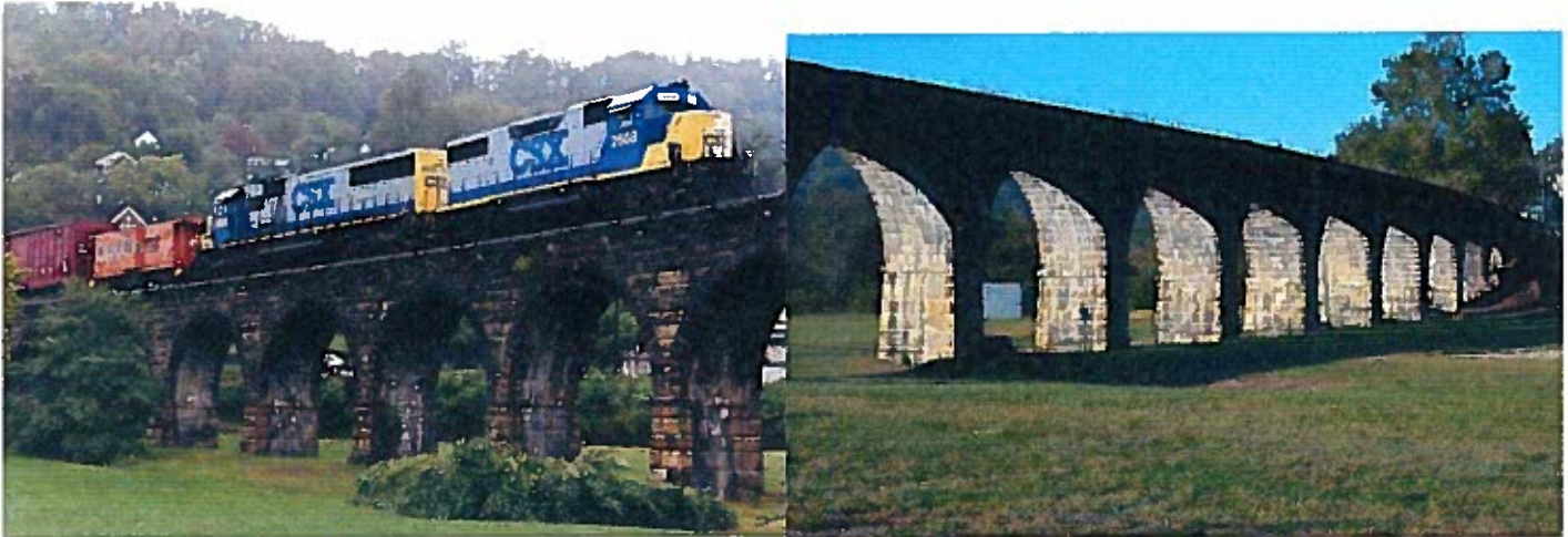
The last locomotives to pass east over the Viaduct on the Newark Subdivision in September, 1996. Photo Daniel Frizzi, Jr.
